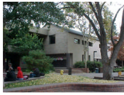
Delta Community College Administration Building
